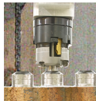
Boiler tube membrane overlay removal and bevel.
